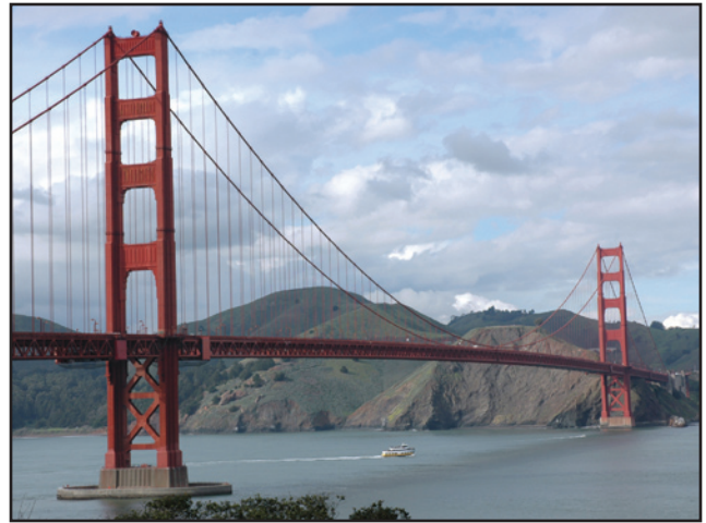
Golden Gate Bridge
