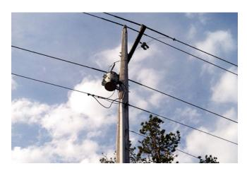
Fig. 11.18. Three-phase to three-wire residential system connected via a step-down transformer. From the pole transformer, the residential power system serving two houses is run down the pole underground. Cape Cod, MA.
